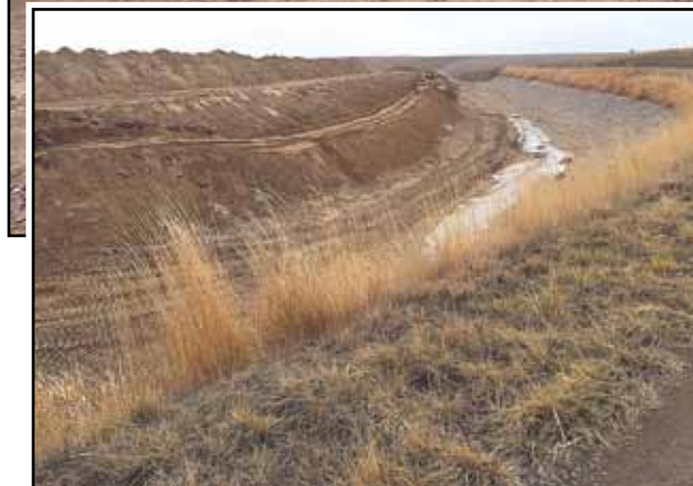
Machinists Union members are widening a 45-mile stretch of the canal that will deliver surface water to farmland. Below just some of the equipment used on the project.
