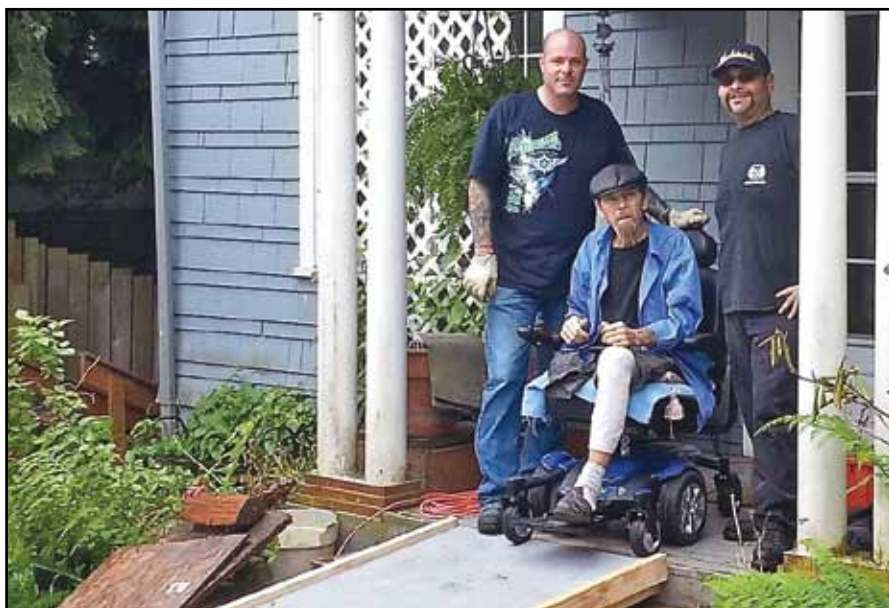
Paul Schubert and Adrian Camez built a wheelchair ramp in Everett.
